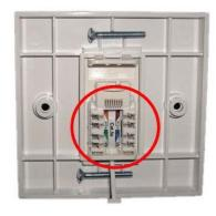
Terminate to "4" & "5". Solid BLUE goes to 4 & BLUE/WHITE goes to "5". For best speeds keep the number of bends to a minimum & make the extension as short as possible. Do not pinch the cable with clips or staples. The RJ45 socket accepts RJ11 & RJ45 plugs (the same as filtered faceplates).
